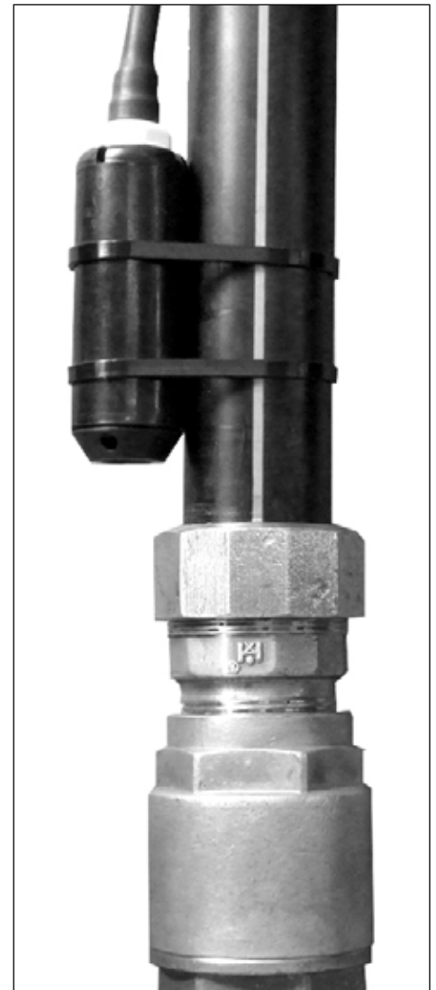
Figure 8: Low-water probe installed in the standard position, for a pump that is positioned vertically
